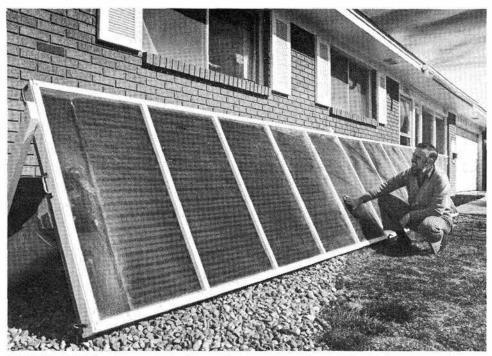
ROSS YINGST checks out his solar collectors. Note duct at lower left through which cool air is blown into the collectors, heated, and circulated back into the house through the greenhouse.
